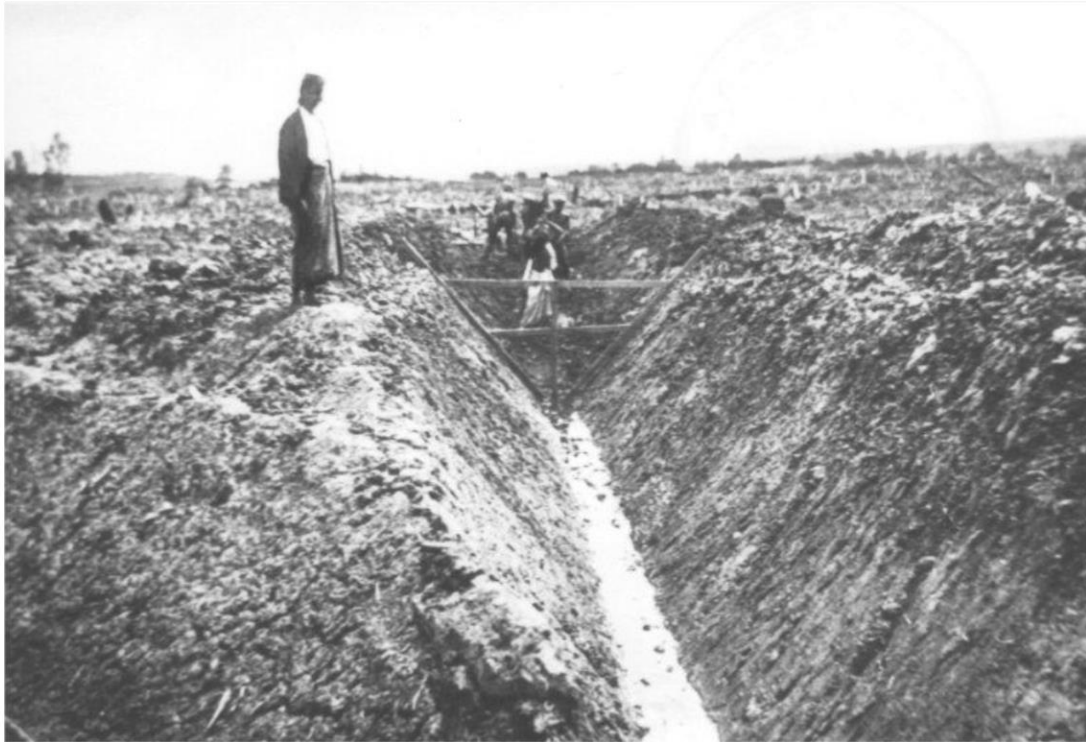
Photograph 2. Labourers excavating a five-foot deep drain on an unidentified coconut holding in Malaya
